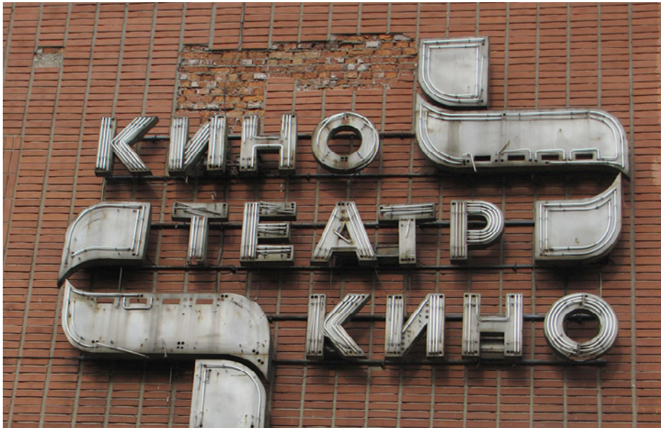
Figure 8: The peeled-off tile cladding of the cinema "Sovremennik" (built after a serial project in 1971), imitating exposed brick, reveals the real brick wall beneath. Source: dariuss, https://dariuss.livejournal.com/500994.html
