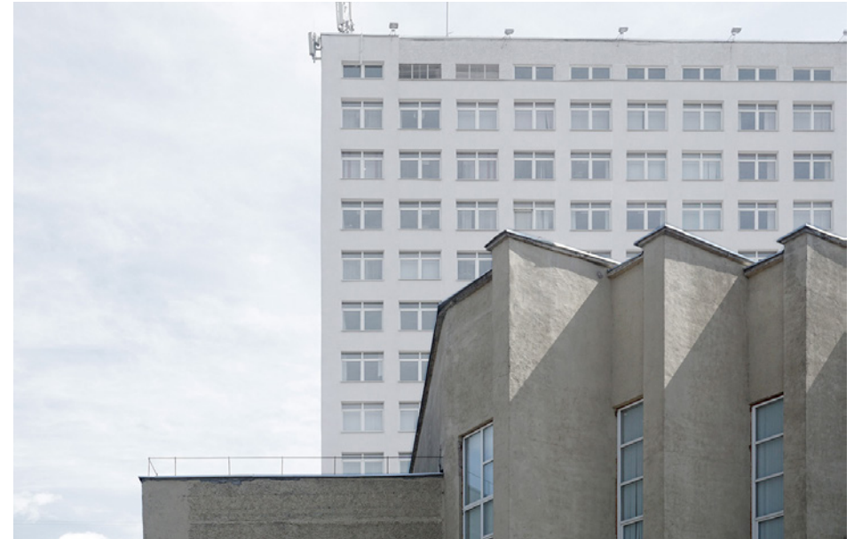
Figure 5/6: Institut Minskproekt, architect L. Pogorelov (1975) The office high-rise, initially grey, emanates the renovation whiteness. The granite-sand-finish of the meeting hall extension still withstands to a certain grade, absorbing the white paint. Source: Author
